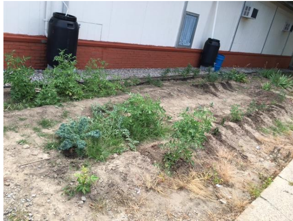
Photo 9: barrels to collect rain water from roof downspouts at St Luke's, water collected to irrigate the vegetable garden. Soaker hose coming off the rain barrels is visible.
